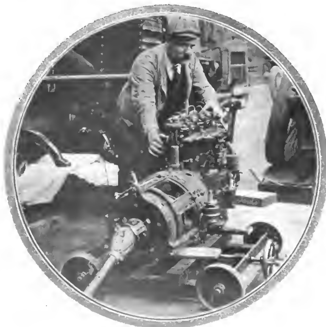
Power unit for a long train of luggers
